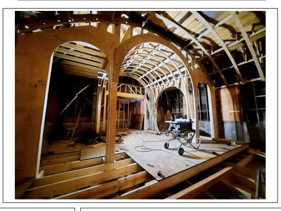
The build is coming along nicely. The plumbing, heating and electrical are all completed. After they are inspected, the insulation goes in and the drywallers close up the walls.
